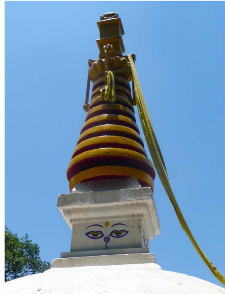
A metal brace holds the crest jewel to the finial. The finial is in need of rebuilding and all stone will be properly cleaned of cement plaster and oil paint.
